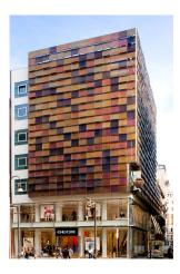
"Breathing Building Geox" is the building above the Geox store in Milan. It is covered with 734 inox steel panels that can be opened with different inclinations, letting the building "breathe" natural air and supporting in a green way the building's air-conditioning system.
